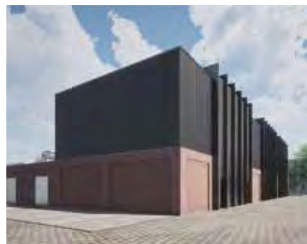
Transformatorstation IJburg, Amsterdam
